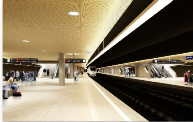
The new Löwenstrasse through station
